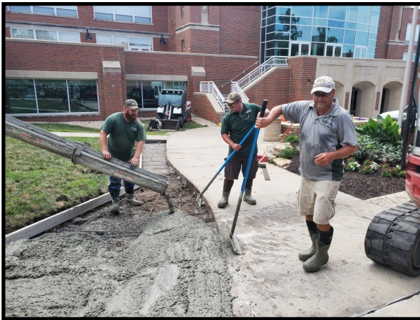
Cody Hoepker, Corey Adwell, David Atkins, Concrete Work
